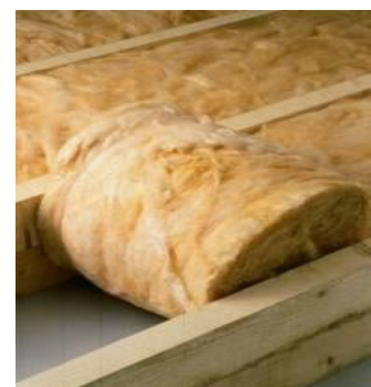
Installing loft insulation
