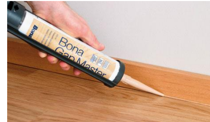
Sealing a gap by a skirting board
