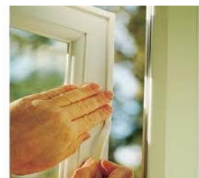
Installing draught stripping
