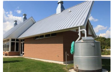
Example rainwater harvesting system
